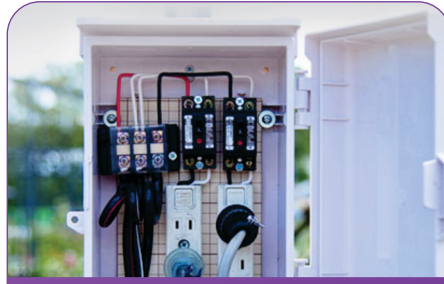
Power Distribution Board
