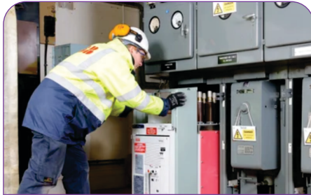
Retrofitting Services & Maintenance Activities Onsite
